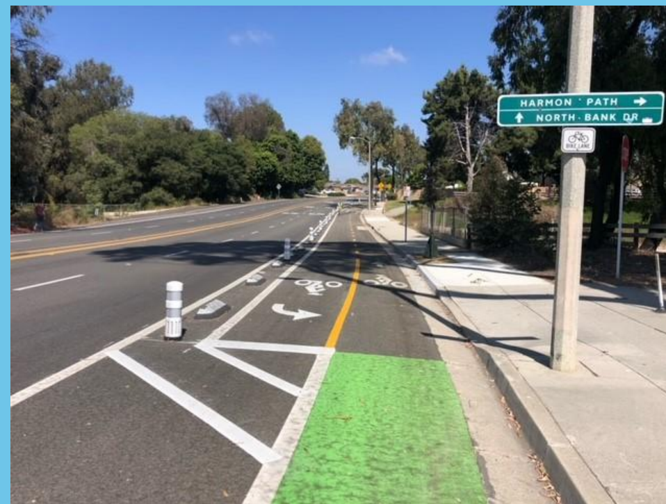
Bristol Road at Johnson Drive Existing
